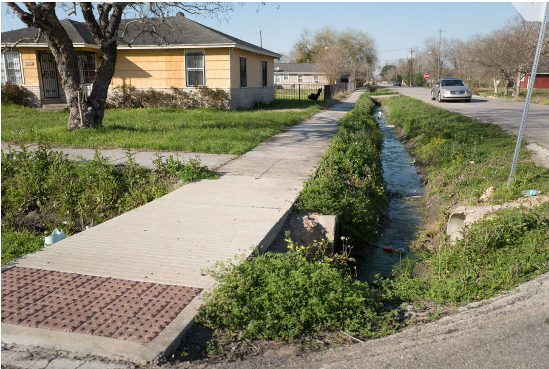
An open ditch drain in a Houston neighborhood
