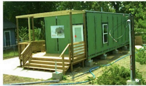
The core takes the place of a FEMA trailer and houses family while waiting for the rest of the home to be built.
