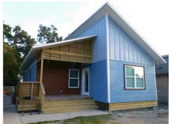
Pre-built panels go together to assemble the temporary “core” house.
