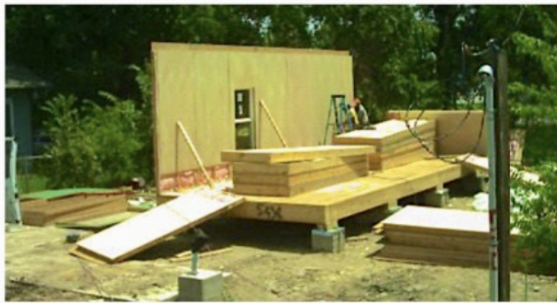
Pre-built panels go together to assemble the temporary “core” house.
